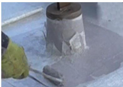
Local reinforcement to stanchion
