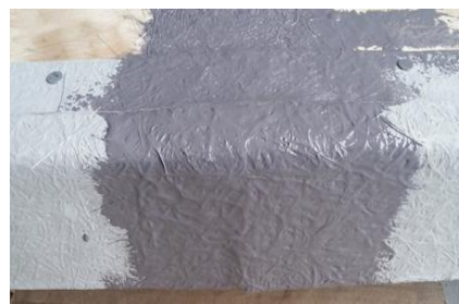
Double reinforced trim joint
