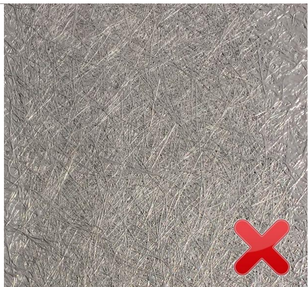
The first coat applied with too little resin or the matting not worked enough, with fibres still straight in appearance
